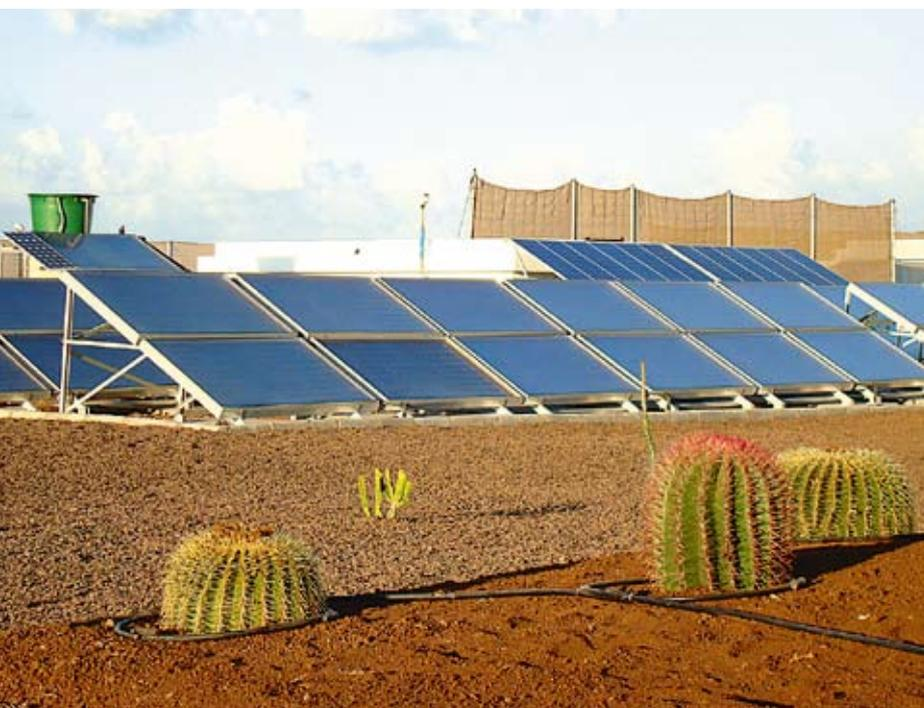
On the Spanish island of Gran Canaria, German researchers from the Fraunhofer ISE set up a membrane distillation system driven by solar thermal energy in 2005. It delivers up to 1,800 litres of drinking water per day.
